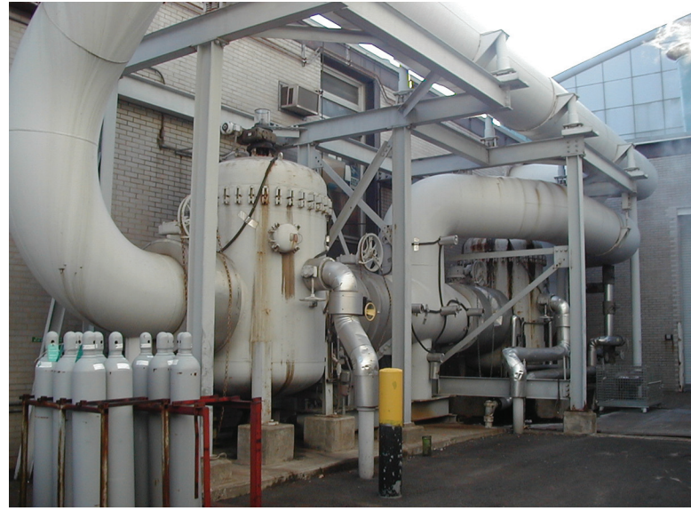
Eaton Model 2596 automatic, self-cleaning strainers have been delivering 15 years of uninterrupted service at JFK airport.
